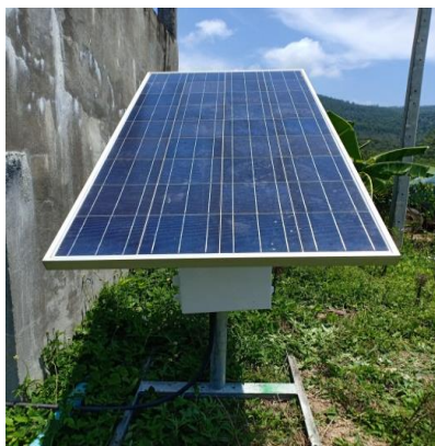
(b) Systems of watering cassava crop by using solar through smartphone.
